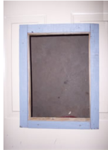
Installed door trim kit.
